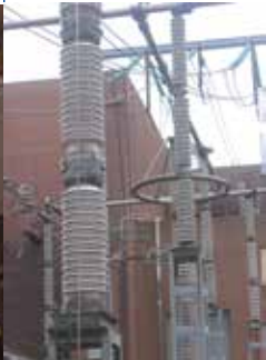
High Voltage Insulator cleaning
